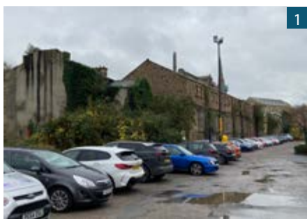
Existing car parking area.
