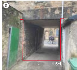
Ginnel (2.4m wide) connecting courtyard behind Stonewell to St Leonard's Gate vehicle route.
