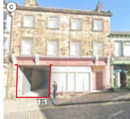
Ginnel (2.5m wide) connecting courtyard behind Stonewell to Moor Lane.
