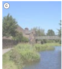
Towpath looking north to Shaw Street iron footbridge (1882).
