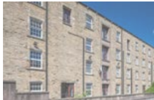
Industrial revolution: White Cross Mill, pictured above and far left (top), Lancaster's first steam-powered mill (1802). Former Springfield Barracks: 1856, Grade II listed, pictured far left (centre).
