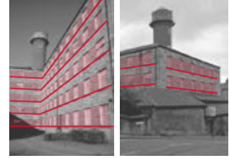
Moor Lane Mill South: Landmark building part of historic mill complex. Simple detailing further emphasises extremely regular horizontal layers.
