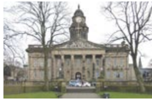
Civic: Town Hall (1909), Grade II* listed city-wide landmark. Edwardian Baroque style, rich carved details. 2 and 3 storeys, pedimented 11 bay entrance elevation. Sandstone ashlar, slate roof.
