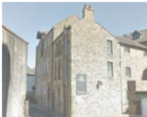
18th C warehouses, Dye House Lane
