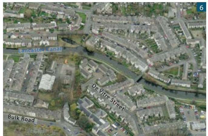
Aerial photo showing the dense residential area to the north-east of the site.
