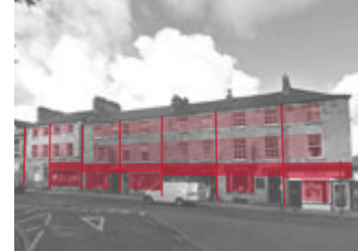
Dalton Square west side: Late 19th century ground floor timber shop fronts form strong horizontal plinth on top of regular vertical glazed bays. Three storey, two bay former residential buildings (Georgian).
