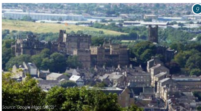
Key strategic view from Moor Lane, the Castle should be visible from this point.
