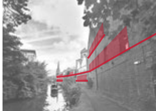
Towpath looking north from Penny Street Bridge: Long low building line, 2-3 storeys, limited detailing leaves emphasis on how windowline echoes the towpath.
