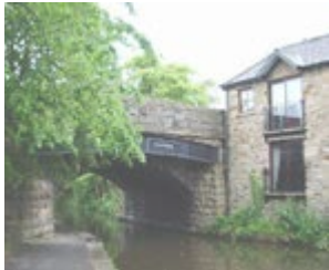
Nelson Street Bridge
