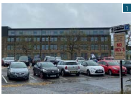
St. Leonard's Gate car park.
