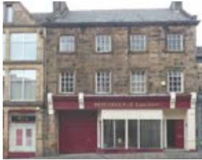
Listed home and shop front, Moor Lane
