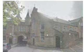
Former Baptist Chapel and White Cross Mill gatehouse: Chapel built in 1872, integrated into the Mill complex in 1894, and new gatehouse built (1899) creating a Mill entrance near Penny Street Bridge.
