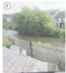
Denis Street looking south to canal and Shaw Street footbridge. Only rear elevations and rear windows face onto the canal.
